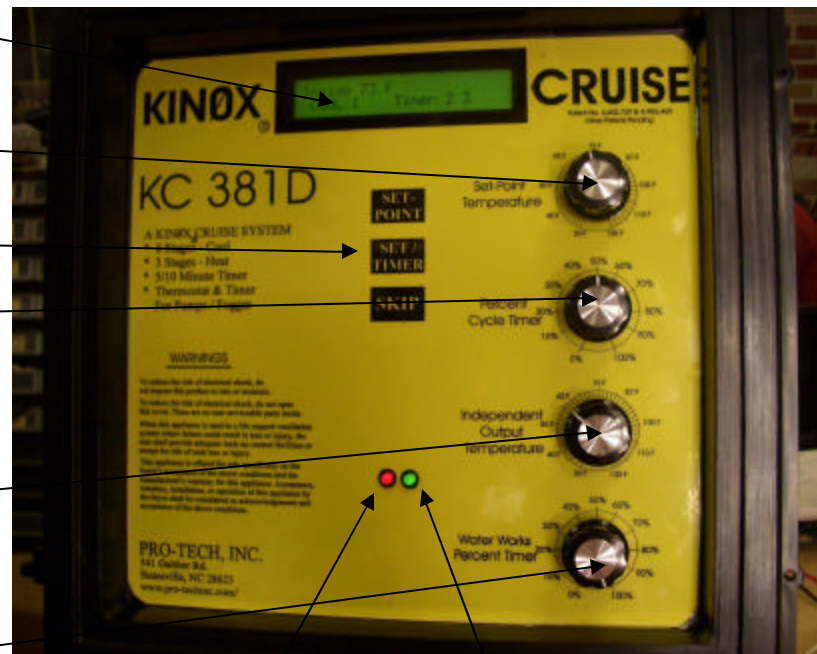
Water Works Cycling
